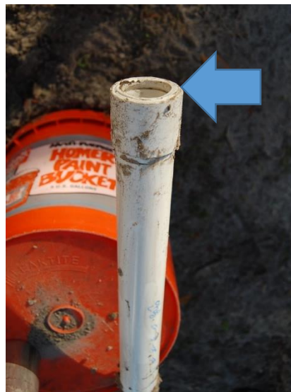
Figure 37. Failed PVC Adapter on Well #5
