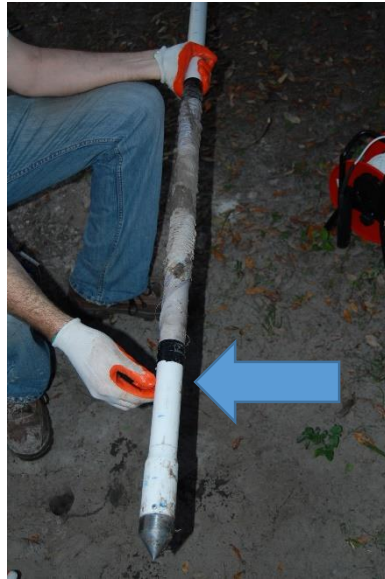
Figure 40. PVC Pipe after Drilling Well #7
