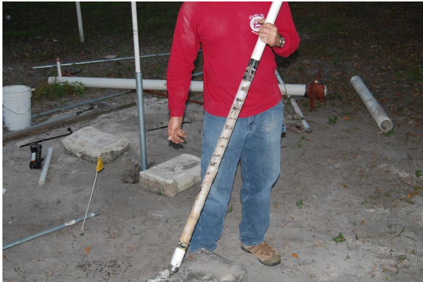
Figure 42. PVC Pipe after Drilling Well #9
