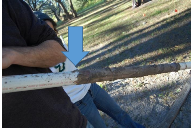
Figure 36. Failed Screen on Well #5
