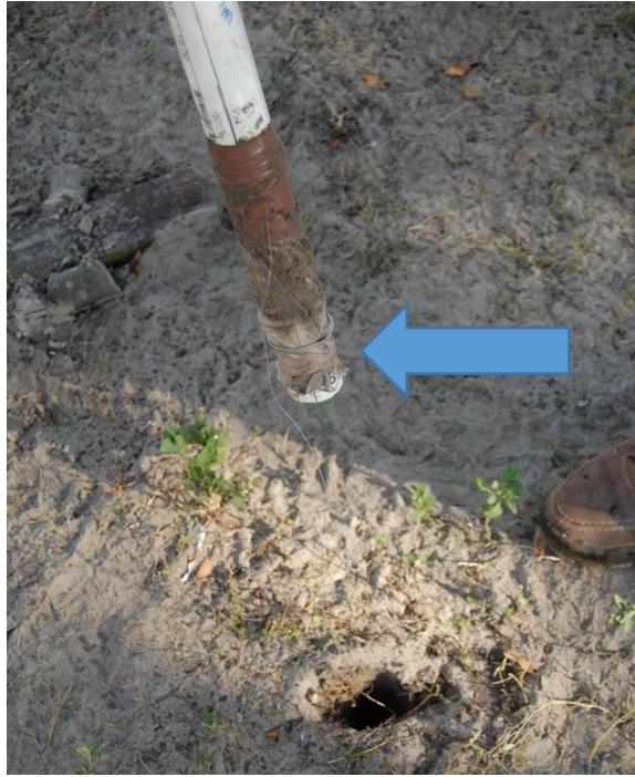
Figure 34. Break in Pipe for Well #3
