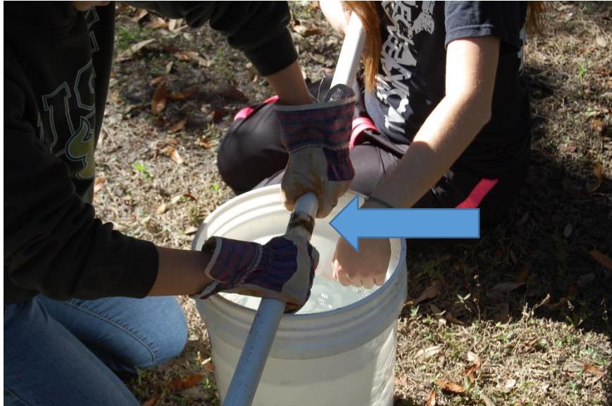
Figure 10. Belling Out a PVC Pipe
