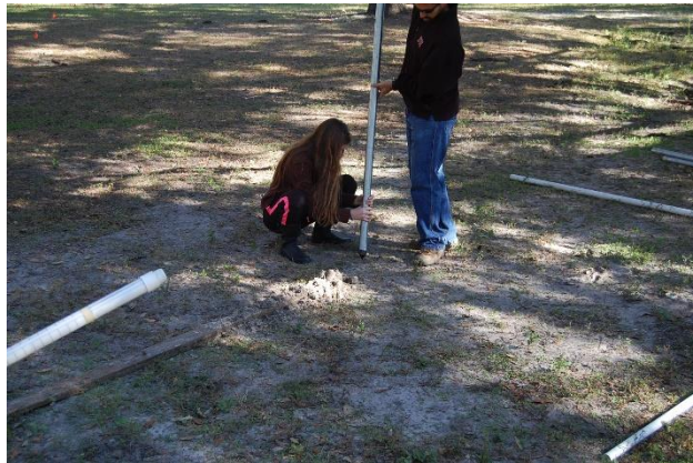
Figure 19. Installation of Cased System
