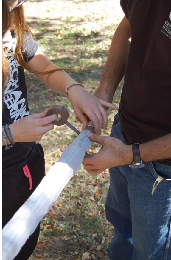
Figure 22. Preparation of the Riser Pipe
