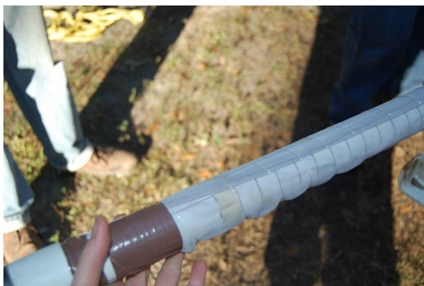
Figure 23. Completed Preparation of Wellscreen
