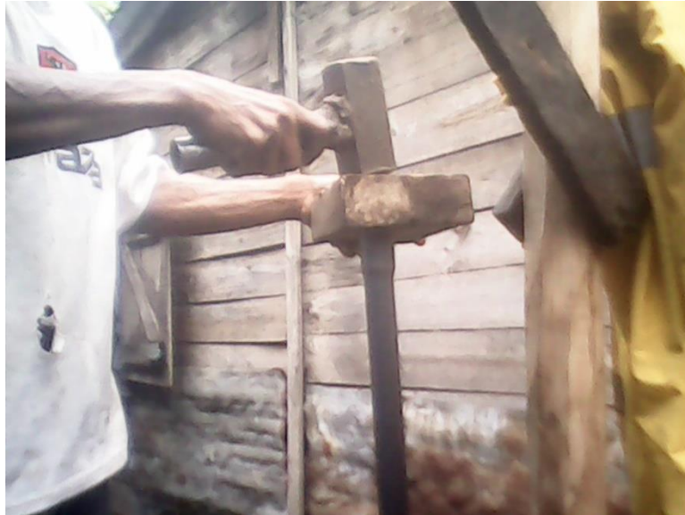
Figure 32. Hammering on PVC Pipe
