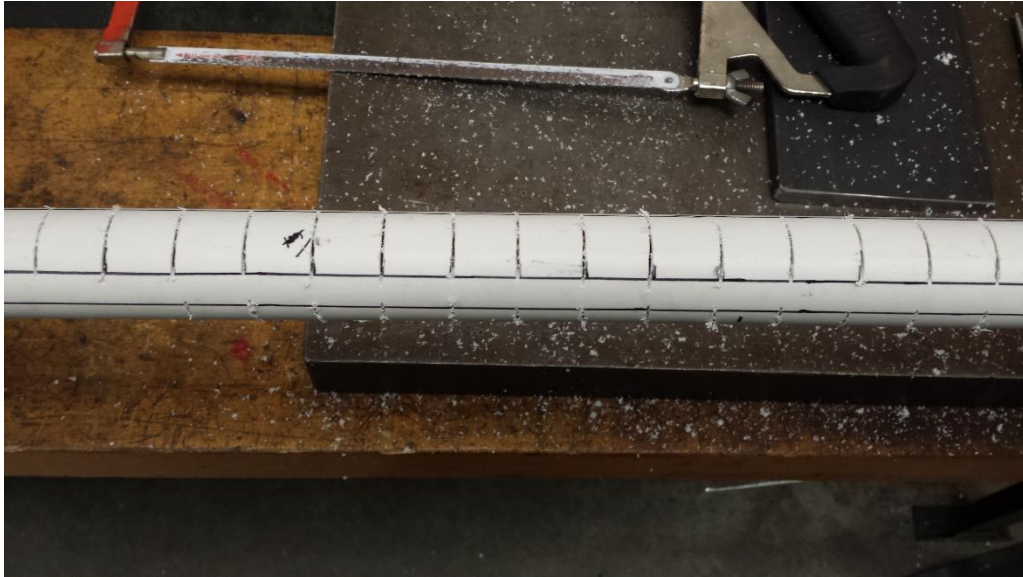
Figure 13. First Method of Screen Cutting
