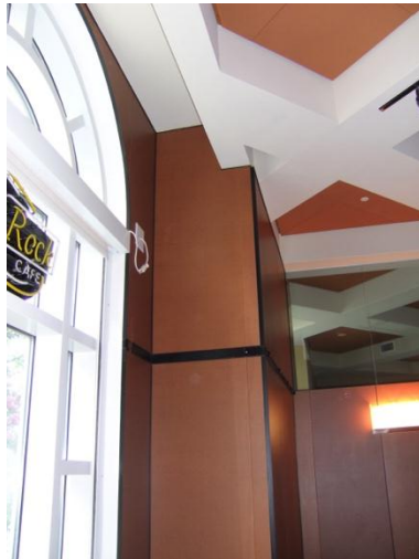
Figure 2: Wall Paneling that extends outwards
